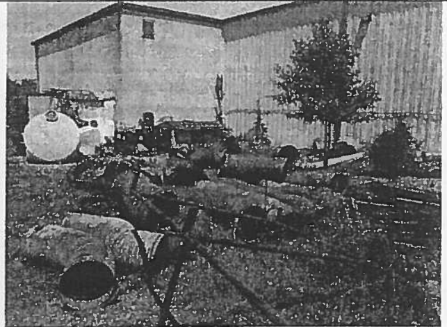
8. West side of building, dirty oil tanker suction piping
